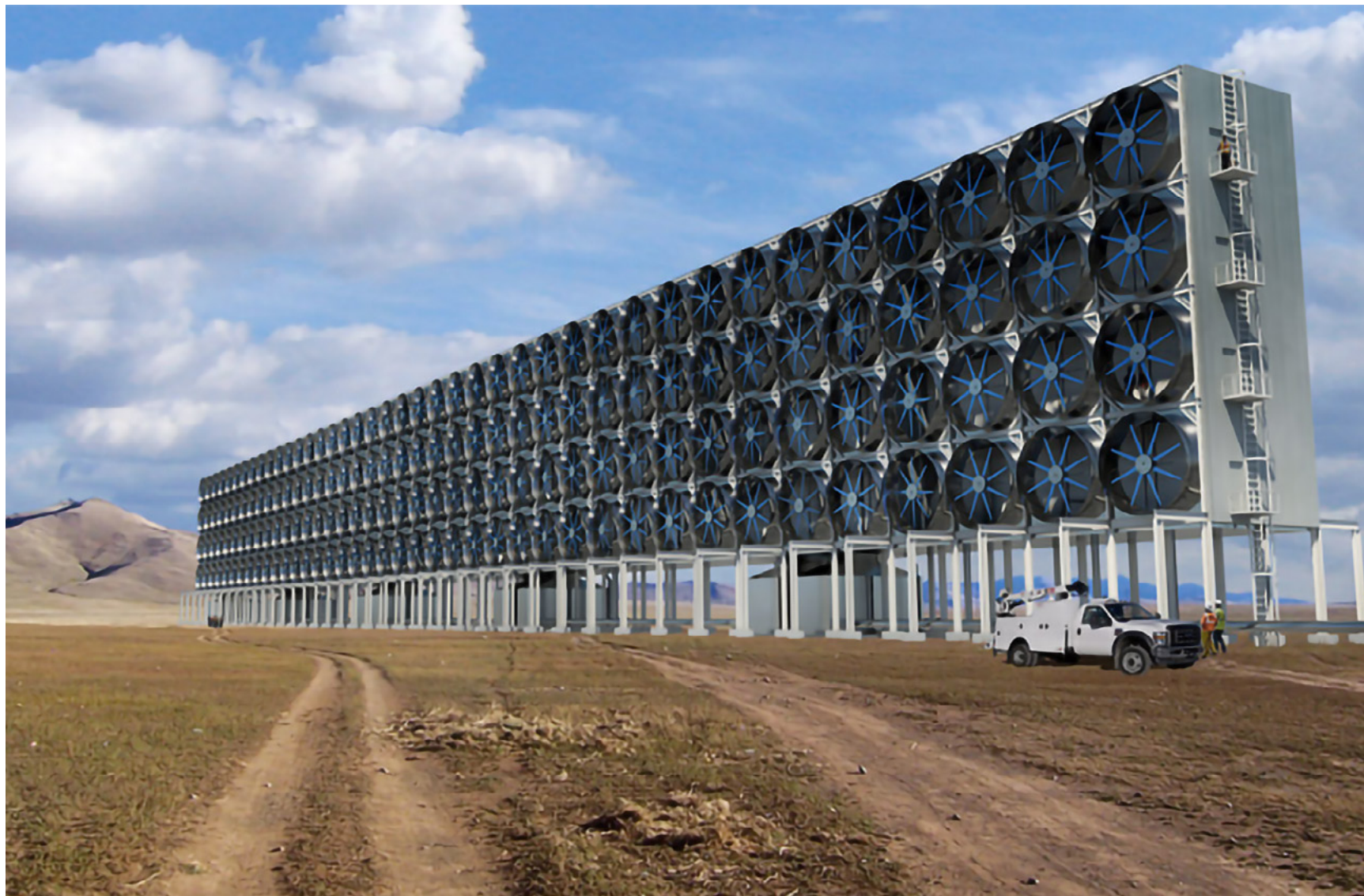
Banks of fans blow air through a CO 2 -capturing solution in this rendering of a DAC plant.
